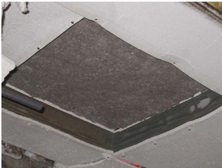
Exposed Side After the Fire Test
